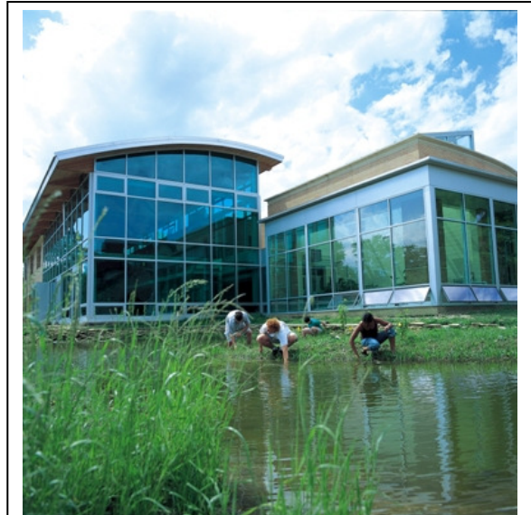
The Adam Joseph Lewis Center for Environmental Studies was one of the first and most innovative green buildings on a college campus when it opened in 2001. It helped launch the green building movement and its innovative systems have since inspired green buildings in many other locations and settings. With over 150 environmental sensors installed throughout the building and landscape, the AJLC's data monitoring and display system provides a unique opportunity to visualize in real-time the flows of energy and cycling of matter that are necessary to support the built environment.
