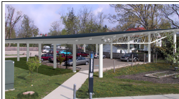
The installation of a solar parking pavilion adjacent to the existing photovoltaic (PV) array on the roof of the innovative Adam Joseph Lewis Center for Environmental Studies makes Oberlin College the home of the largest PV array in Ohio, with a total rated production of 159 kW. Sunlight collected by the panels on the 8,800-square-foot pavilion roof is transformed into a maximum of 100 kilowatts of electrical energy, bringing the center's total rated production (based on peak theoretical output under ideal conditions) to 159 kW, equivalent to the amount of energy needed to power nearly 15 single-family homes.
