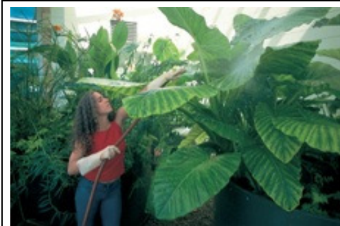
The Living Machine processes wastewater into reusable grey water via the natural cleansing methods that occur in a wetland—plants, bacteria, protozoa, and other aquatic microorganisms are used to clean and condition the water for reuse. It is located in the Adam Joseph Lewis Center for Environmental Studies, and it is operated by a group of about 10 students.
