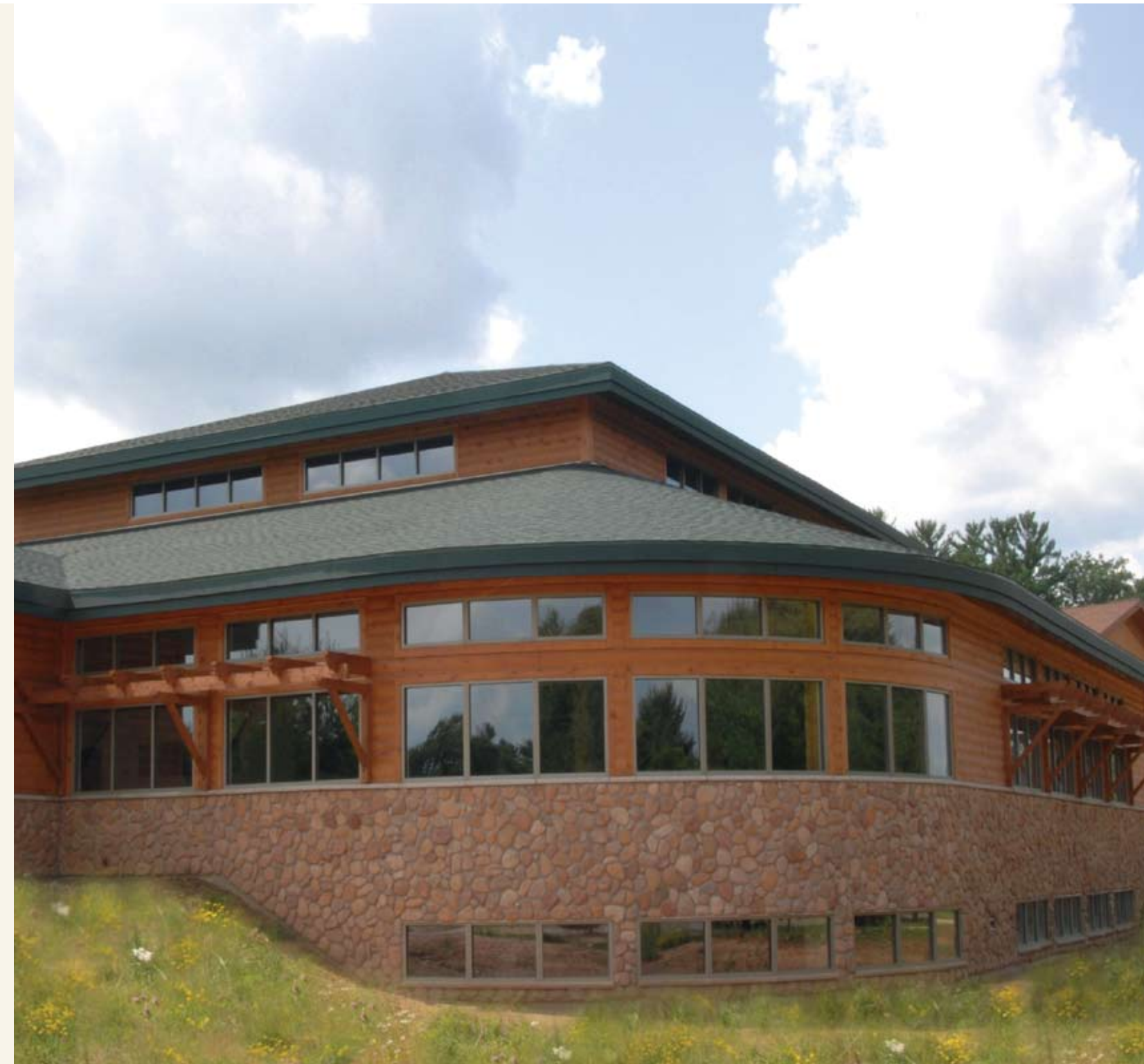
The newly constructed library at College of Menominee Nation utilizes passive solar design and ground-source heating and cooling. (Photo: D. Kakkak)
