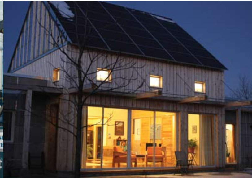
The Unity House, a zero-carbon LEED Platinum building at Unity College
