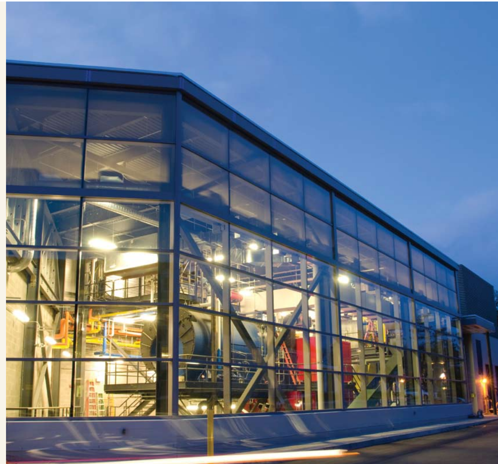
The new biomass gasification plant at Middlebury College will replace a million gallons of heating oil and reduce carbon emissions by 40% per year, a big piece of the college's plan for achieving carbon neutrality by 2016. (Photo: Middlebury College)
