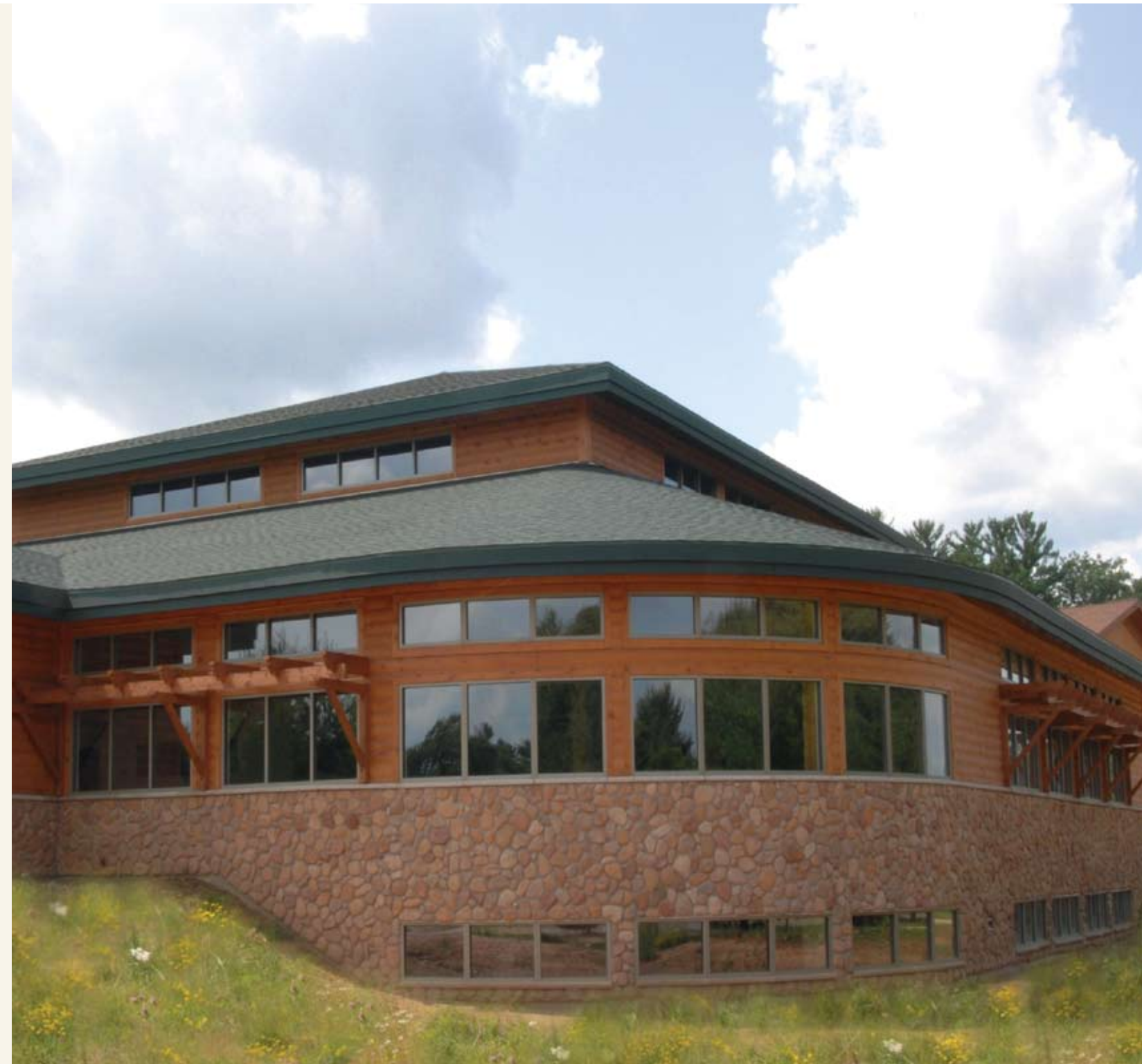
The newly constructed library at College of Menominee Nation utilizes passive solar design and ground-source heating and cooling. (Photo: D. Kakkak)
