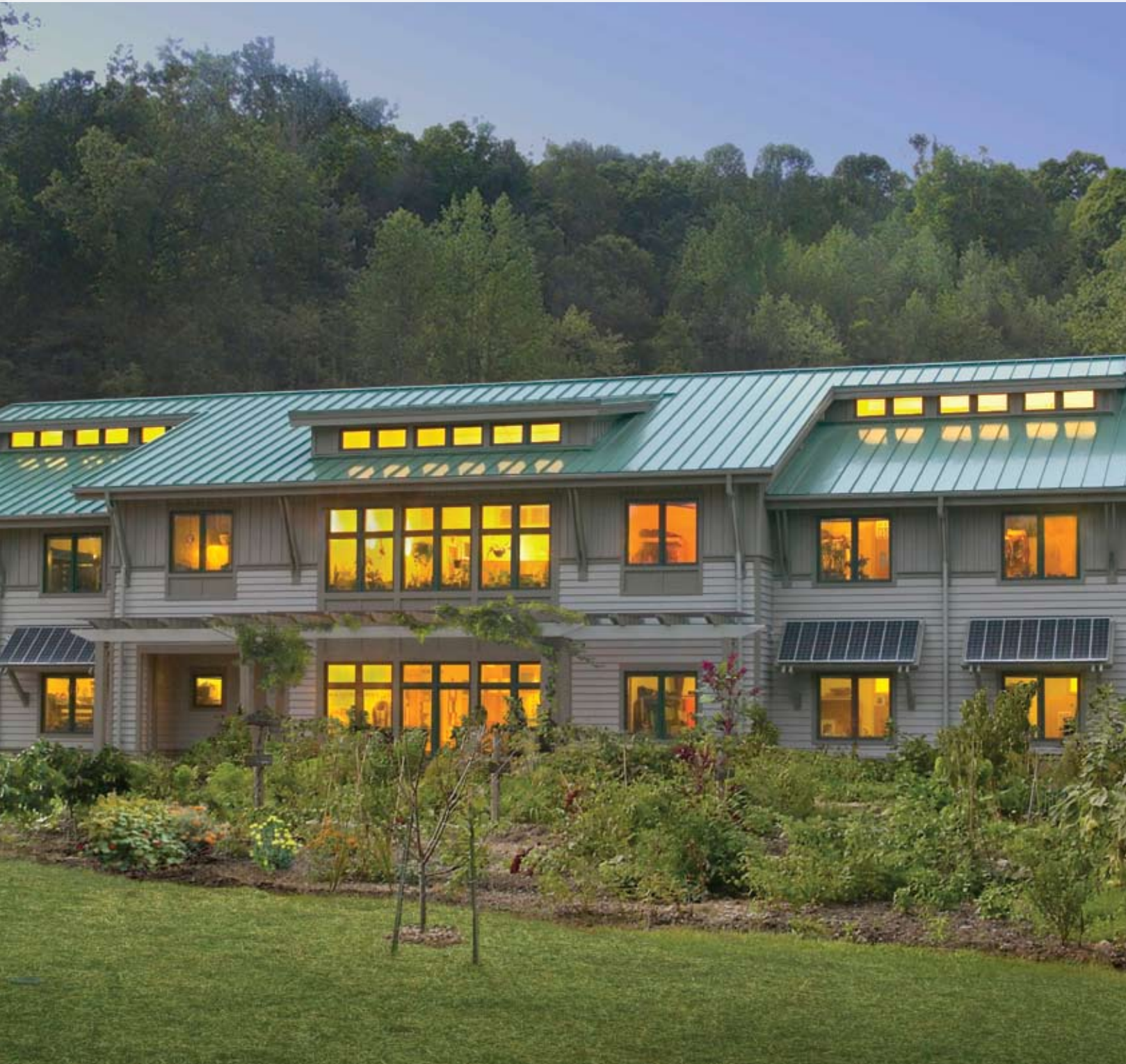
Warren Wilson College's ecoDorm uses one-third the energy of comparable conventional buildings. (Photo: Warren Wilson College)
